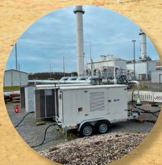
LMF mobile pipeline evacuation units in action
